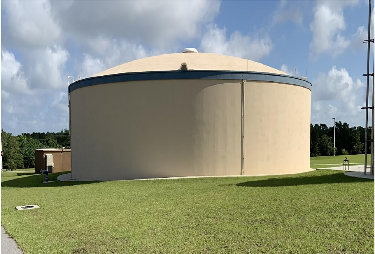
Figure 1 Central Regional Water Production Facility
