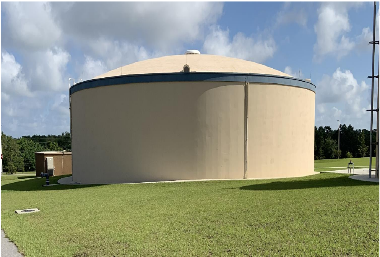
Figure 1 Central Regional Water Treatment Facility
