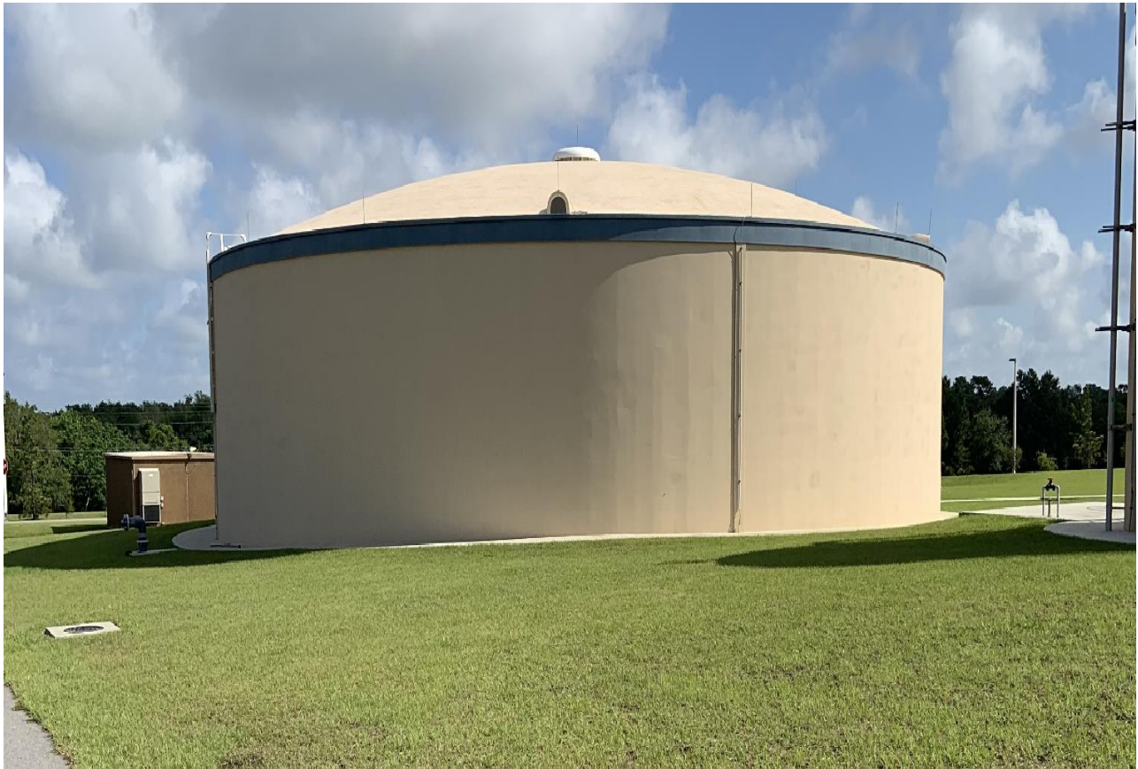
Figure 1 Central Regional Water Production Facility
