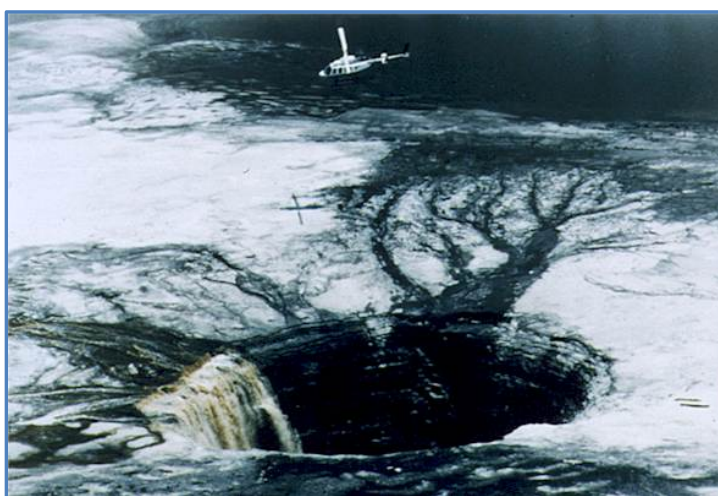
Figure V.47: Sinkhole in Center of IMC-Agrico Waste Stack Near Mulberry, June 1994 Source: www.fluoridealert.org (AP Photo)
