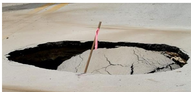
Figure IV.13: Sinkhole/Depression middle of Kathleen Road September 2012; Source: The Ledger
