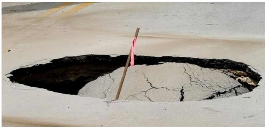
Figure V.27: Sinkhole in Kathleen Road from collapsed pipe
