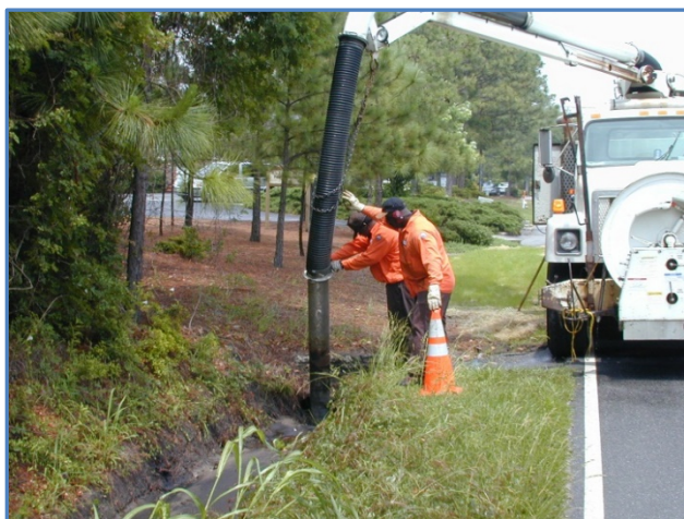
Figure VII.6: Drainage system maintenance
